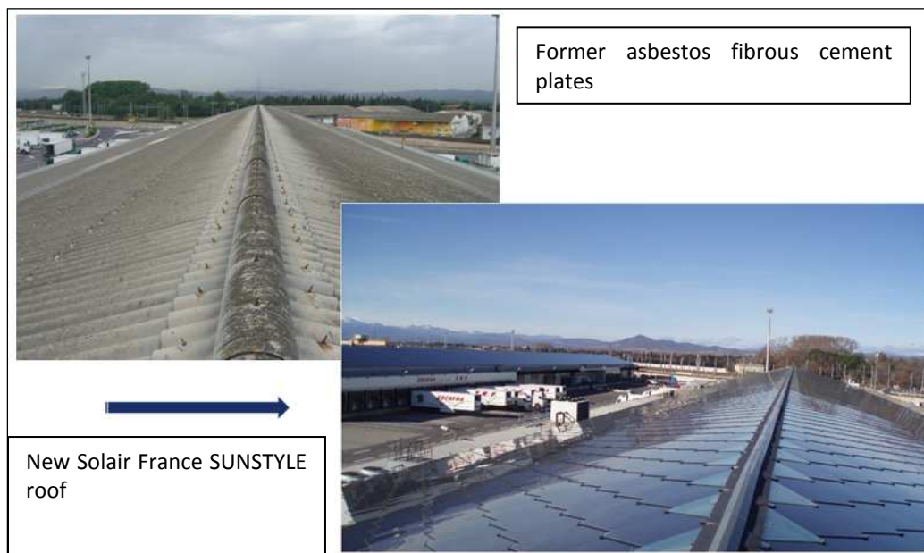
Figure 2: Replacement and renovation of the former roof
